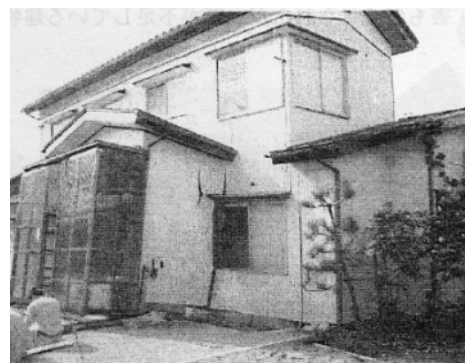
Photo 8 Uneven settlement of wooden house on soft soil caused by earthquake 8)
