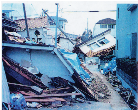
Photo 6 Collapse of wooden house caused by lack of bracing in the first story 6)
