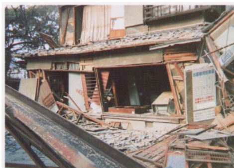
Photo 4 Inclined wooden house without bracing in south side 6)
