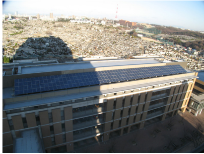
Fig. 14 A shadow on a PV system installed in MEIJO University south building covered with "Tower 75"
