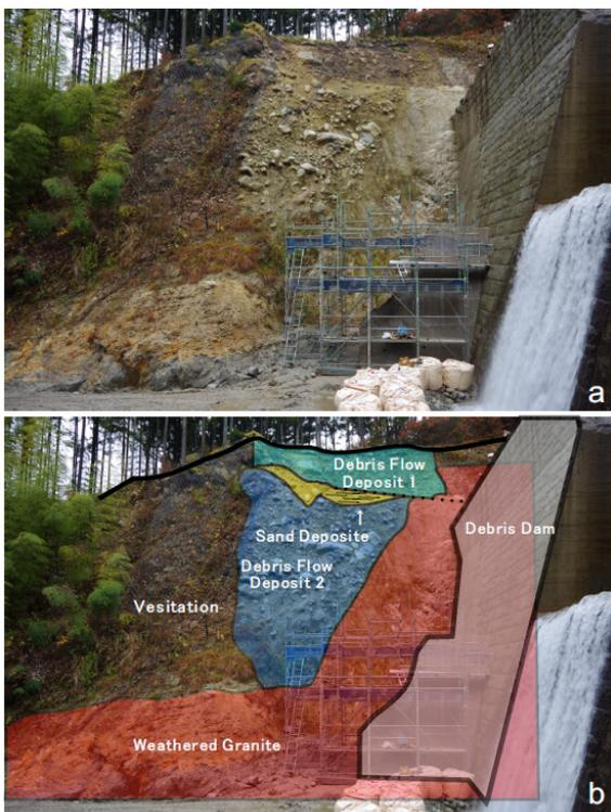
Fig. 6 Geological Outcrop along the right side of Nashizawa Second Debris Dams
